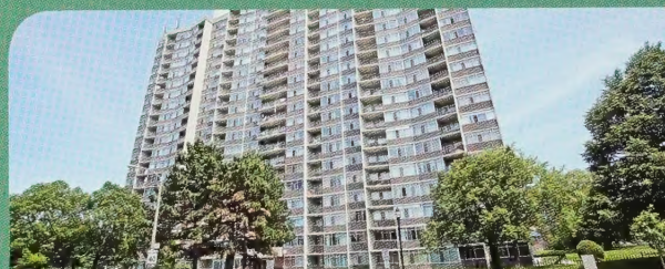
25 Bay Mills Boulevard
